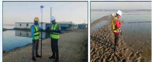
Topographic Survey using CHCNAV i93 at Matarbari
