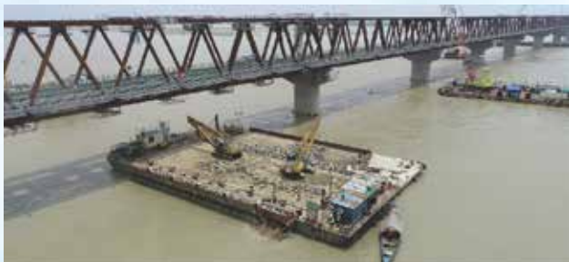
Dumping Berge at Jamuna Rail Bridge
